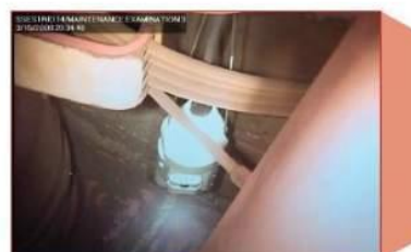
PTZ100 camera head positioned in between section jet pumps at the base of the core shroud horizontal weld.
